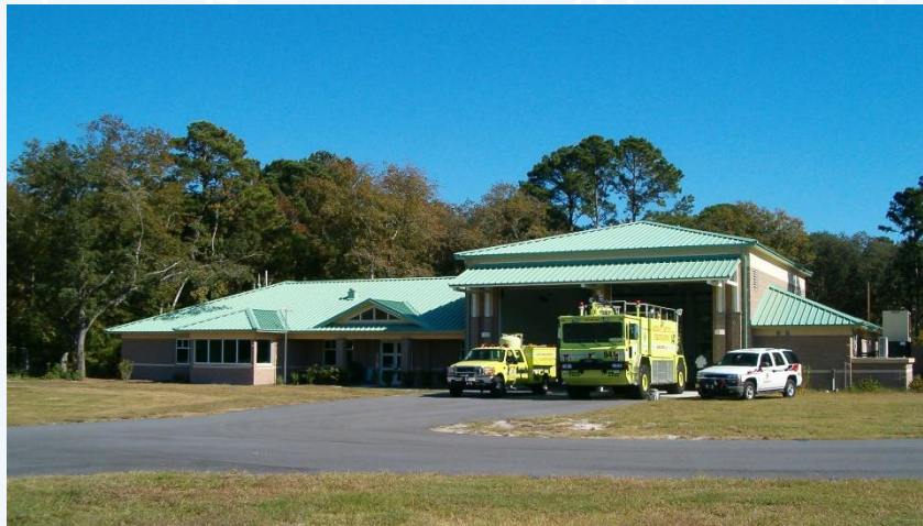
Hilton Head Island Airport Aircraft Rescue and Firefighting Facility
